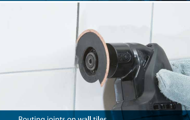
Routing joints on wall tiles
