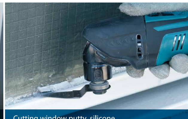
Cutting window putty, silicone
