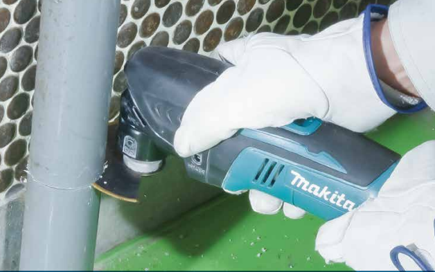
Cutting PVC, FRP pipes
