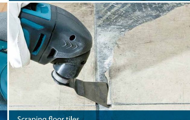
Scraping floor tiles
