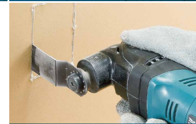
Cutting plasterboards
