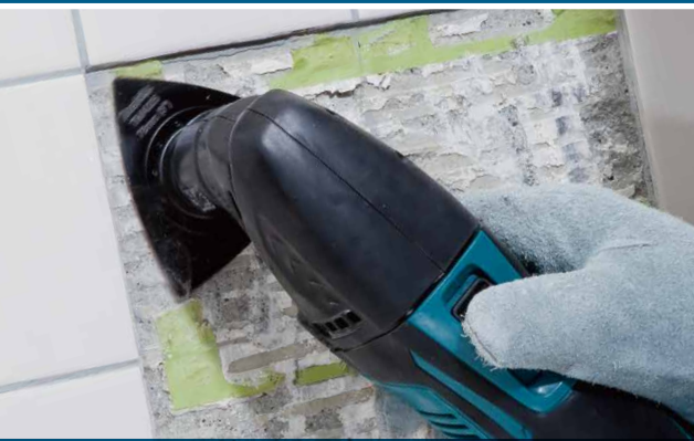
Removing mortar, tile adhesive
