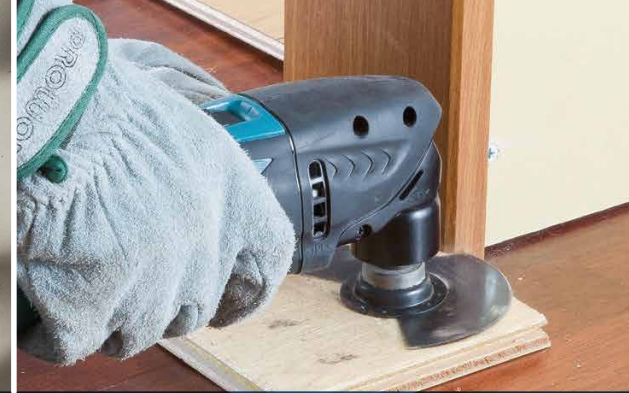
Wood flush cutting
